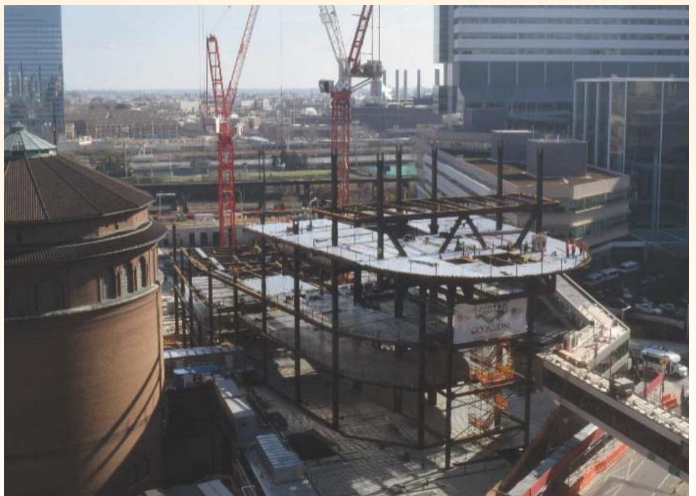
‘New Pavilion’ Hospital taking shape, construction as of February 2018
